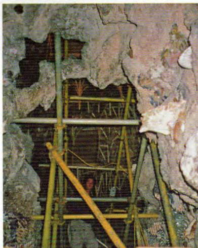
FIGURE 5. Scaffolding for access within the six metre high volume
